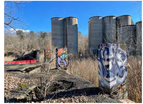
Iron Mountain Cement Silos Penny Coleman
