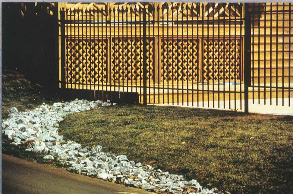
The rock-lined channel shown in this housing development slows the flow of runoff and safely conveys it to a place where it can percolate into the ground.
